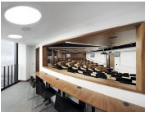
Above and right: Free-hanging rafts and acoustic wall panels in the lecture theatre are micro-perforated to make them sound-absorbent despite having the appearance of solid timber.
